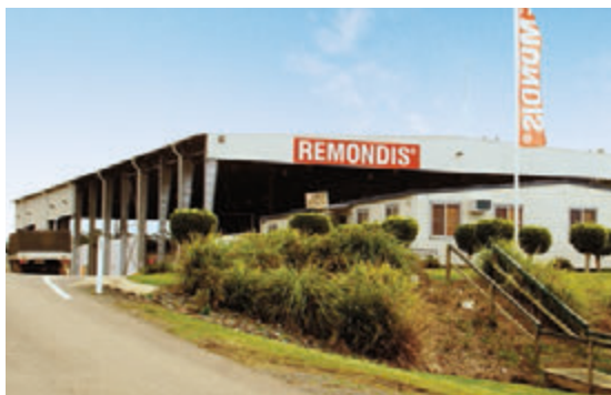
REMONDIS' Mugga Lane waste transfer station
