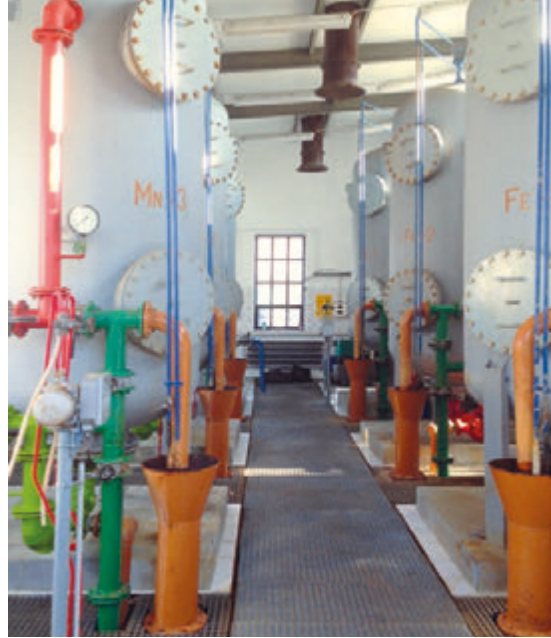
The waterworks in Wyszogrod have been upgraded
