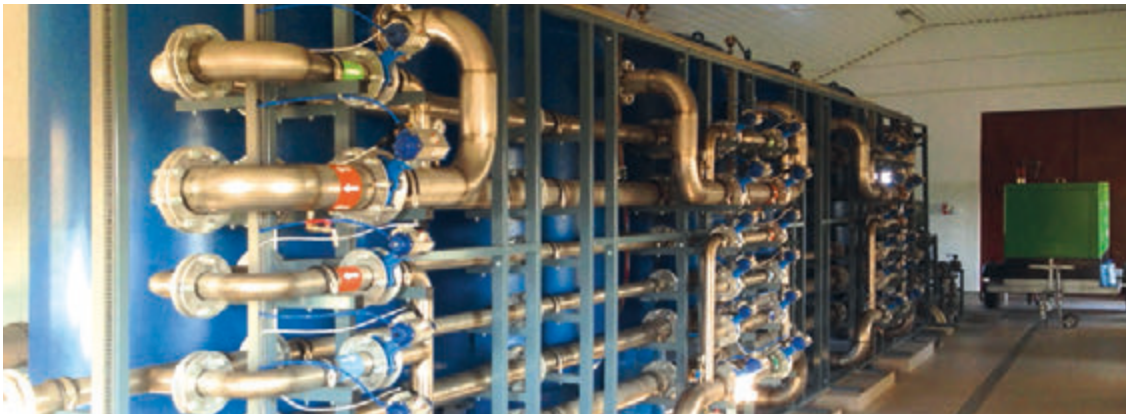
Kobylniki also uses state-of-the-art water technology now
