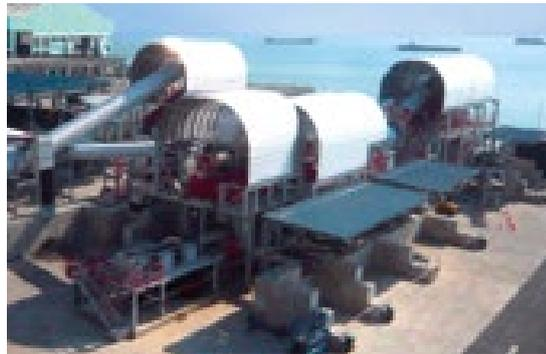
from Singapore's four household waste incineration plants and to recover any metals contained in the ash. A good 90 percent of the ferrous metals and over three quarters of the valuable non-ferrous metals, such as aluminium and copper, will be able to be recovered and recycled – even the really small pieces like paper clips and bottle caps.
