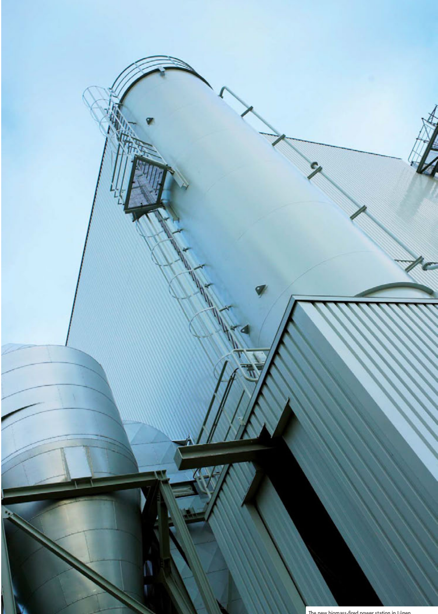
The new biomass-fired power station in Lünen
